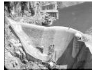
Ataguía o presa auxiliar 1952: EASTMAN 35 SAFETY FILM PANCHROMATIC (25D H91590)
